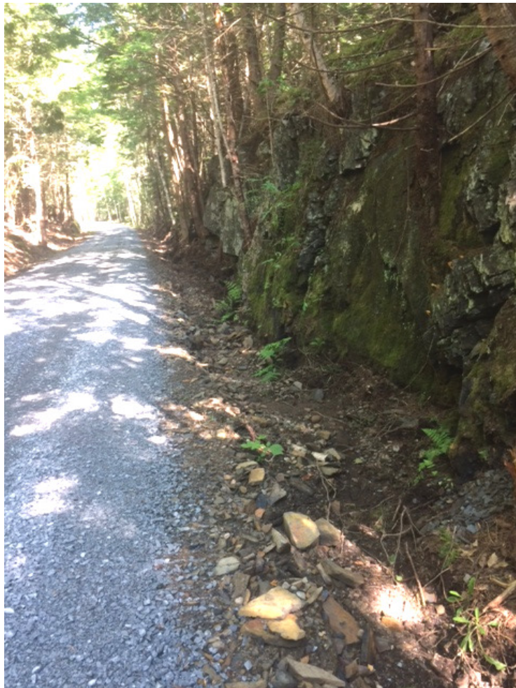
New surfacing and ditching at Salmon Run to Wentzell Rd
