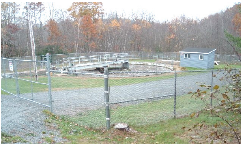
New Germany sewage treatment plant November 2005
