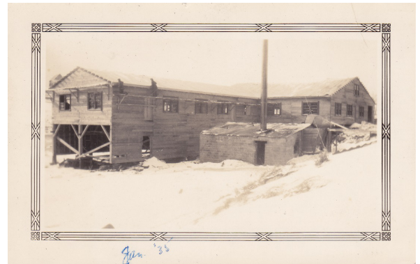
The only known photograph of the new mill under construction in 1935.
