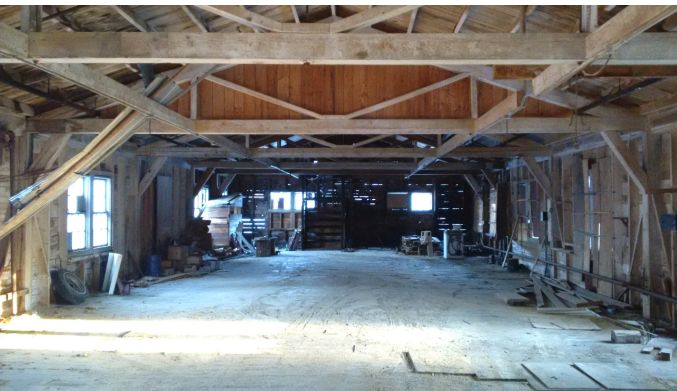
A current view of part of the top floor of the factory.
